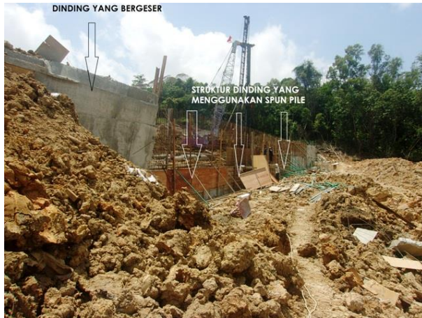
Gambar 1.5 Dinding Penahan Tanah Bergeser
