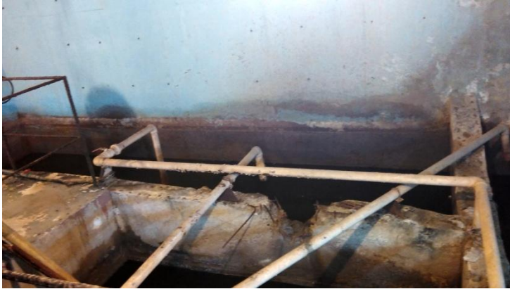
Gambar 3.4 Unit Sludge Tank
