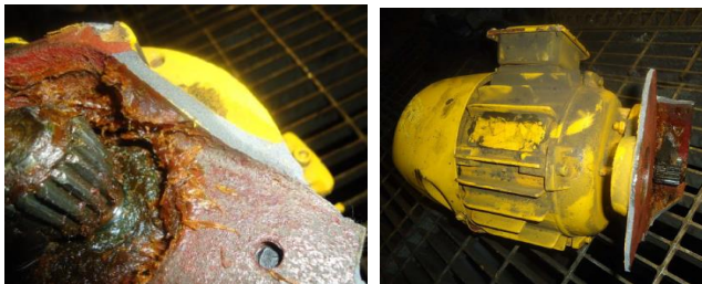
Gambar 1.3 Patahan Housing Motor Hoist
