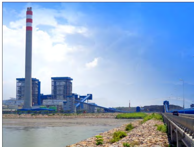
Gambar 1.1 PLTU Rembang (View from jetty)
