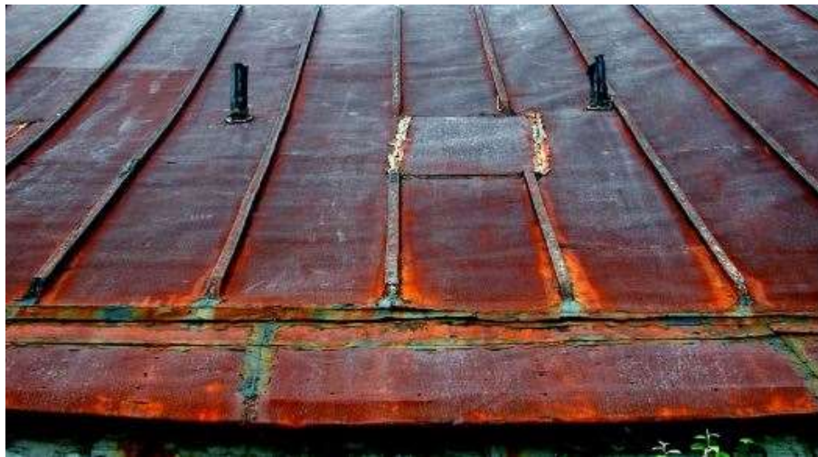
Gambar 2.2 Uniform Attact ( www.corrosiondoctor.org )
