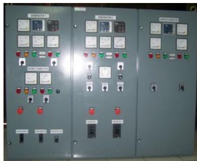
Gambar 2. 4 MSB (Main Switch Board)
