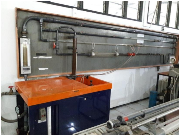
Gambar 3.1. Instalasi sistem perpipaan CUSSON friction loss in pipe apparatus
