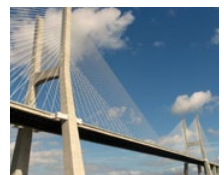
Vasco da Gama Bridge (PT)
