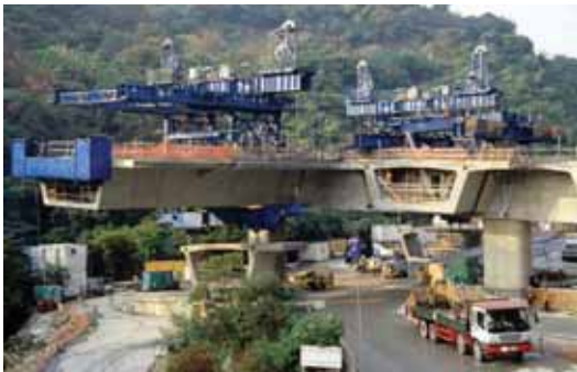
Lai Chi Kok – Hong Kong (2004-2005) 63,000m 2 of deck, 1,771 segments
