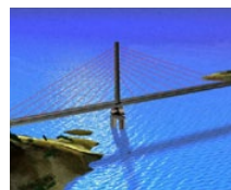
Agin Bridge (TR)
