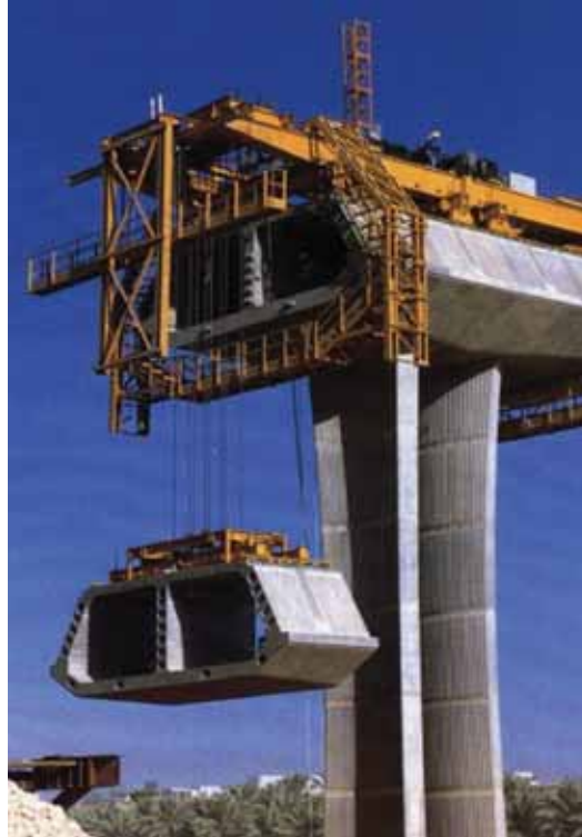
Quarashia Bridge – Saudi Arabia (1989-1990) 12,820m 2 of deck, 143 segments
