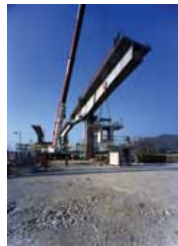
West Rail - Hong Kong (1999-2002) 8,330m 2 of deck, 617 segments
