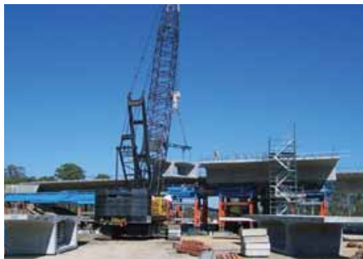
West Link - Australia (2004-2005) 86,000m 2 of deck, 3,013 segments
