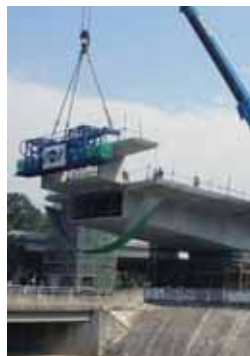
Shatin T3 - Hong Kong (2004-2007) 65,800m 2 of deck, 1,806 segments
