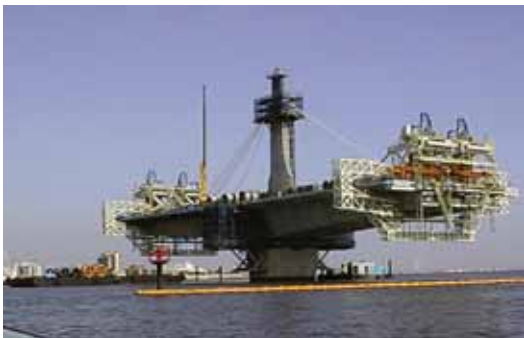
Kisosansen Bridge – Japan (1998-2001) 90,000m 2 of deck, 344 segments
