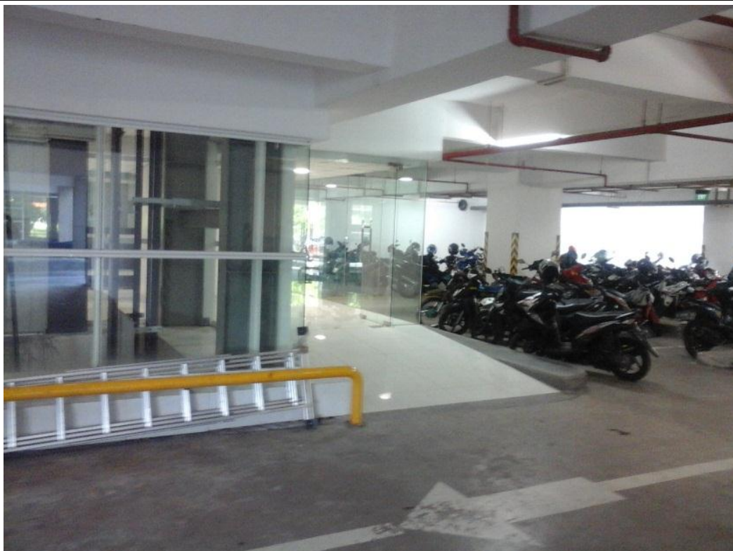
Gambar F.91 Pintu Masuk Gedung Research Center ITS
