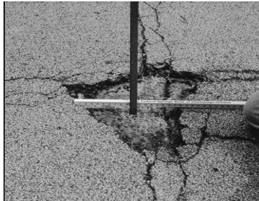
Gambar 2.14 Lubang ( Potholes ) Sumber: ASTM
