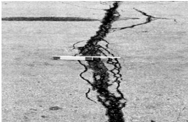
Gambar 2.9 Retak Sambungan ( Joint Reflection Cracking ) Sumber: ASTM
