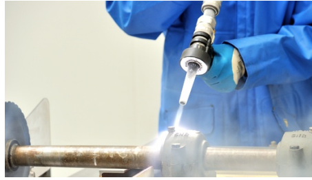
Gambar 2. 13 Proses Dry ice blasting
