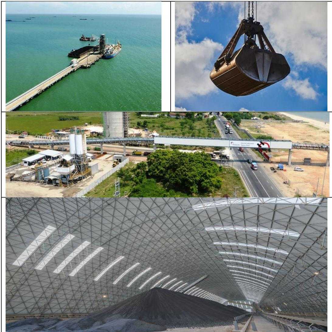
Gambar 4. 2 fasilitas *discharging coal* di jetty area meliputi *grab*, *belt conveyor* dan *dome storage*
