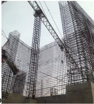
Gambar 10.3 Penulangan Shearwall
