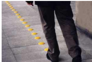
Figure 4.4 Tacdot that guide the user thourough the building
