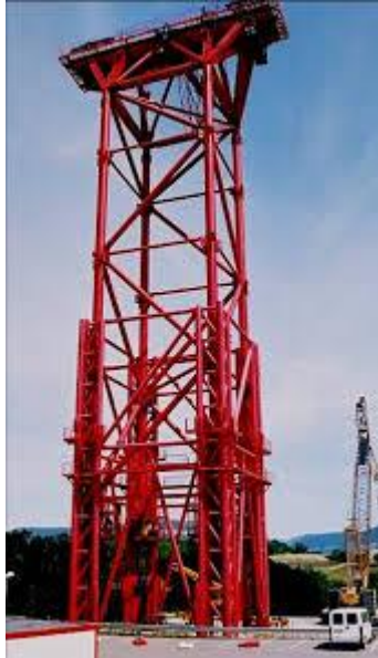
Gambar 9.11 Pemasangan Temporary Tower
