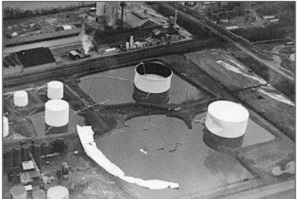
Figure 2. 1 The aerial photo of a split tank remaining and “dented” neighboring tank at right.
