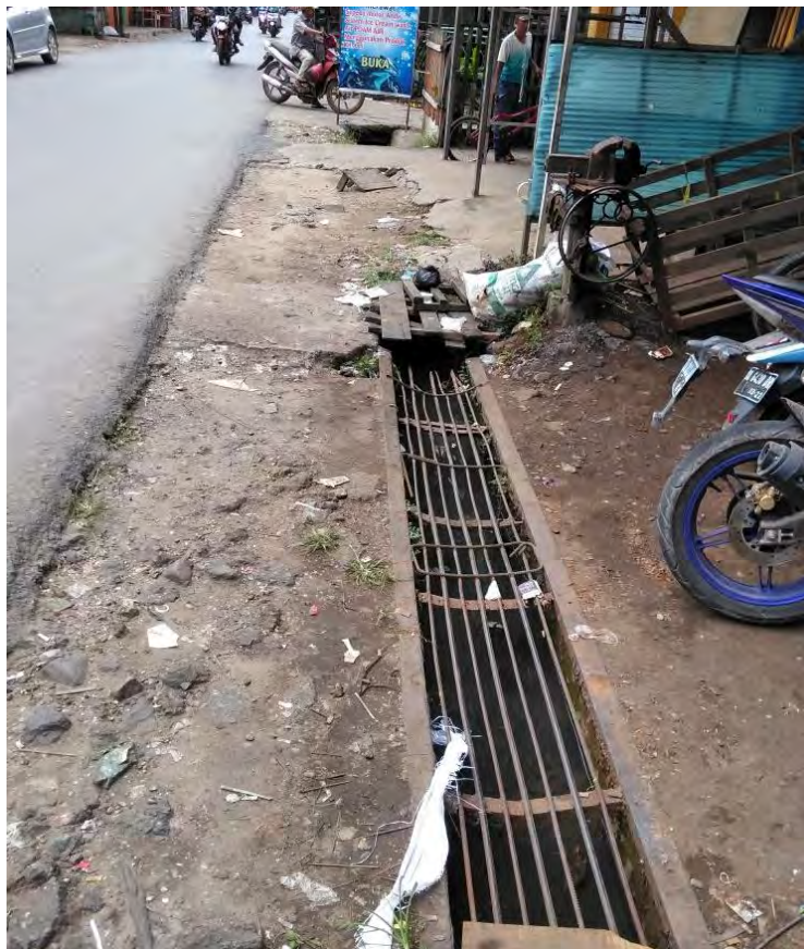
Gambar Lamp 5.8 Kondisi Drainase
