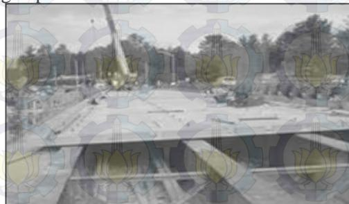
Gambar 2.8. *Full Slab precast*
