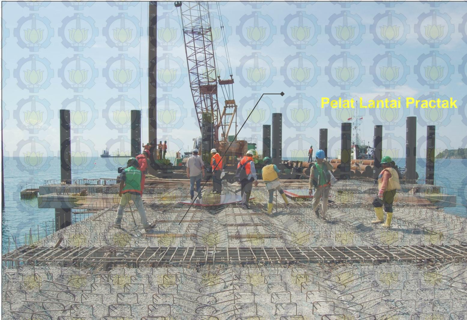
Sistem Pelat Lantai Half Slab Precast
