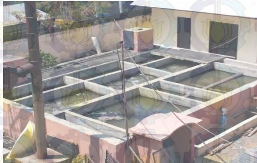
Gambar 3.5 Activated Sludge Rumah Sakit X
