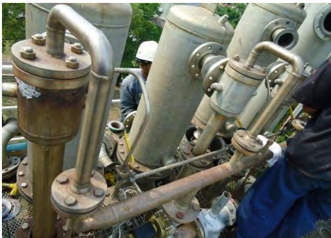
Gambar 4.12. Pengecekan Vacuum Unit
