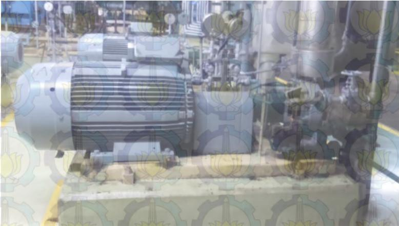
Gambar 2.30 *Low Pressure Boiler Feed Pump*
