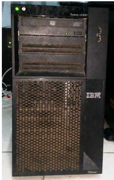
Gambar 4.3 LPSE Web Server
