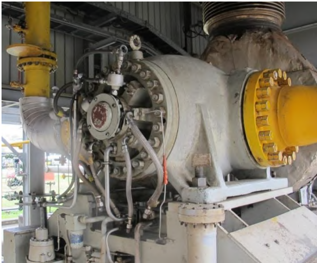
Gambar 3.3 Centrifugal Compressor C-306
