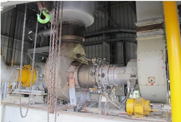
Gambar 3.2 Centaur 40 Gas Turbine by Solar Turbine
