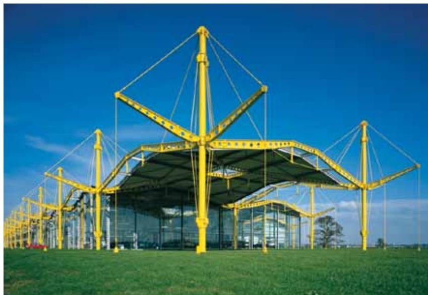
The Renault building in Swindon, recognised as the world's first tensile structure, is supported using the Macalloy Tension Bar System. This building has now been granted grade 2 listed status, due to its architectural significance.
