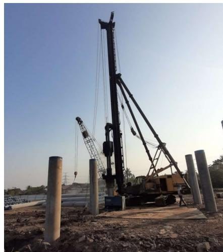
Gambar II.8Pile Drive – Hammer
