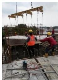
**Gambar 2. 15** Proses Pemasangan *Half Slab Precast*
