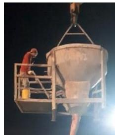
**Gambar 2. 23 Concrete Bucket**
