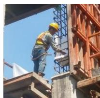
**Gambar 5. 15** Pemasangan *Block-Out Link Beam*
