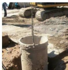
**Gambar 5. 1** Pemasangan *Temporary Casing*
