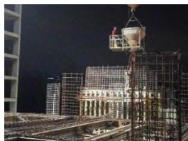
**Gambar 5. 18** Proses Pengecoran *Shearwall*
