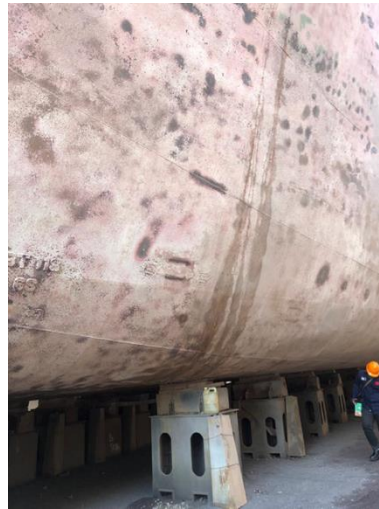
Hasil Sand Blasting
