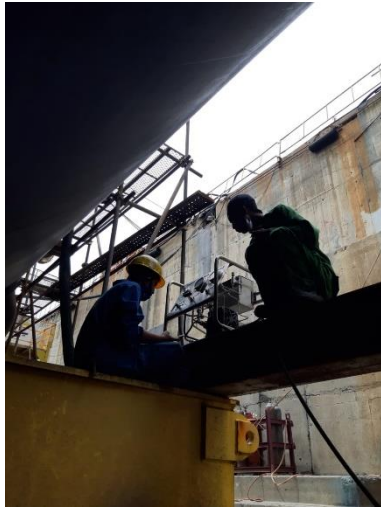
Pressure Test Valve (hydro test) KRI Alugoro (Kapal Selam)
