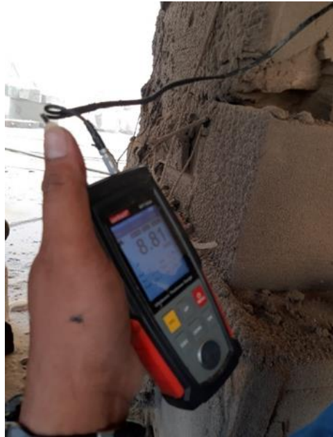
Gambar 5.9 Ultrasonic Gauge Wall Thickness
