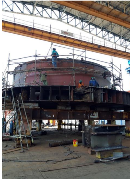
Proses Perbaikan Single Point Mooring
