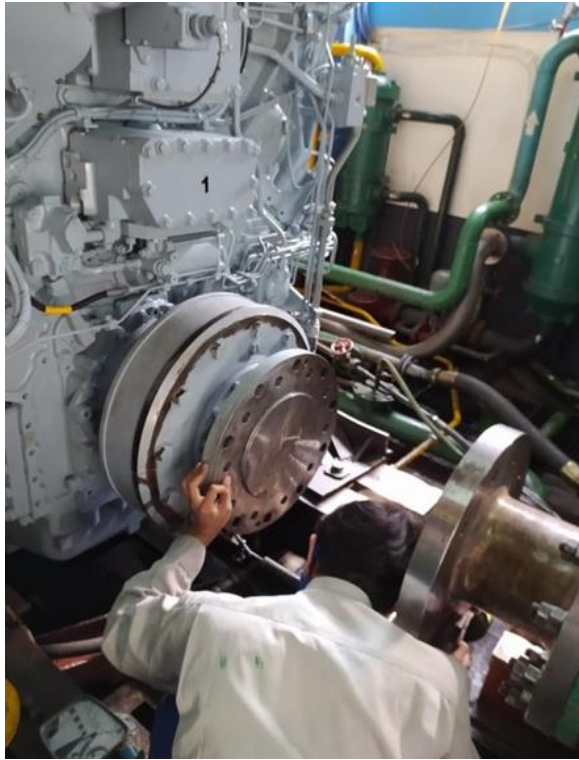
Gambar 3.2 Proses Alignment Engine terhadap Water Brake
