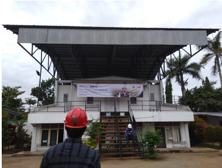
Gambar 2.3. 3 Site Office (Ruang Meeting, Divisi Engineering, dan Divisi Legal)
