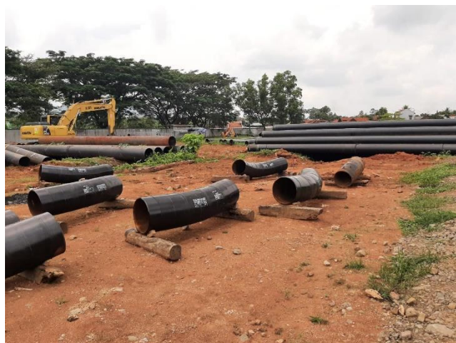
Gambar 2.3. 8 Site Office (Area Bending)
