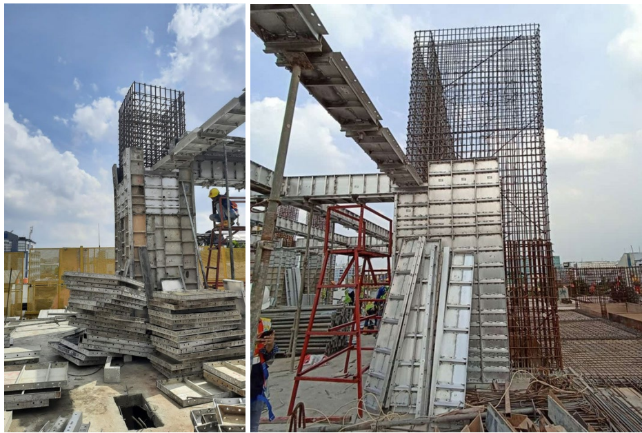
Gambar 6.1 Pemasangan Aluminium Formwork
