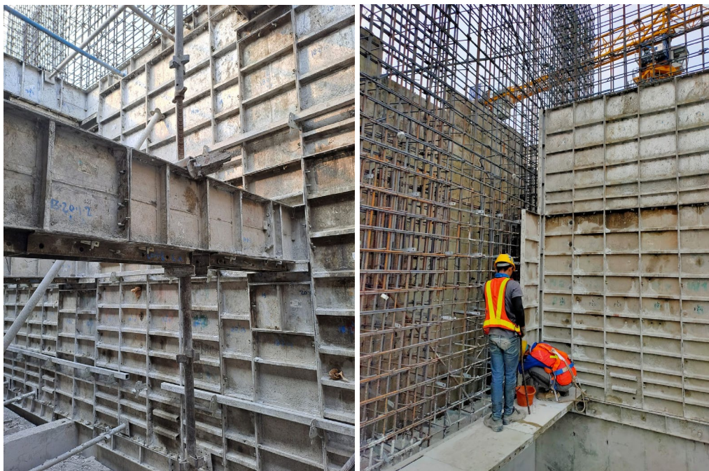
Gambar 3.16 Alumunium Formwork
