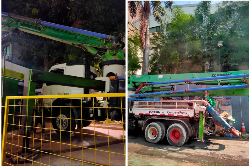
Gambar 3.9 Concrete Pump & Pumping
