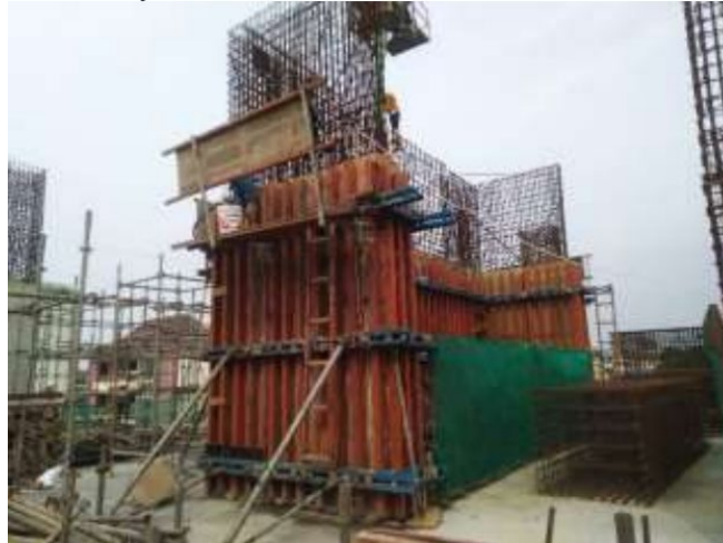
Gambar 3.17 Bekisting konvensional Area Podium
