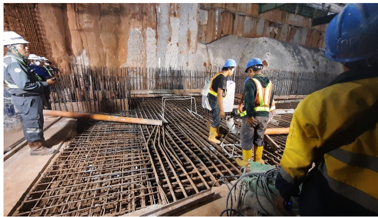
Gambar 5.25 Persiapan Pengecoran Mass Concrete Raft Foundation
