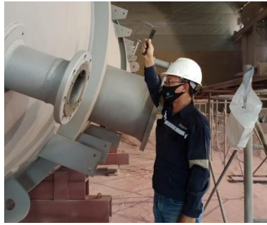
Gambar 4. 5 Proses Quality Control Painting ( Sumber : dokumentasi pribadi )
