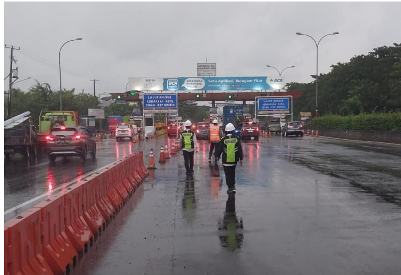
Gambar III.14 Pelaksanaan Inspeksi Heavy Maintenance
