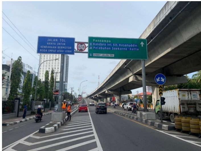
Gambar III.6 Rambu Penunjuk Arah On Ramp Allauddin
