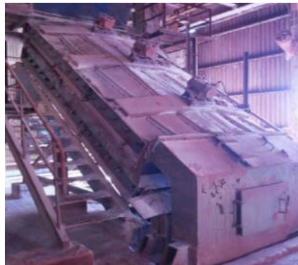
Gambar 4. 6 Over and Fines Screen
