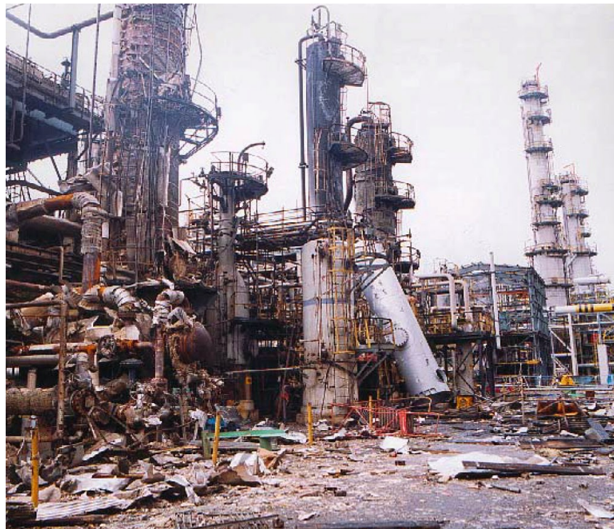
Figure 2. 1 Explosion at The Conoco Humber Refinery (Source: Jonathan Carter, et al, 2006)
