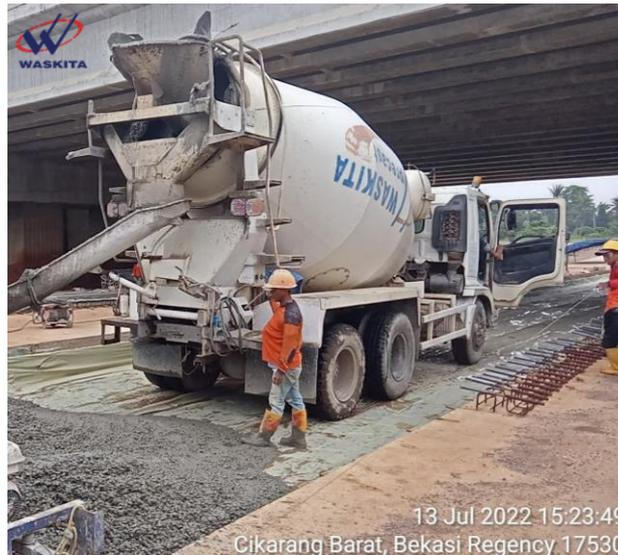
**Gambar 2.5** *Truck Mixer* kapasitas 7 m<sup>3</sup>
