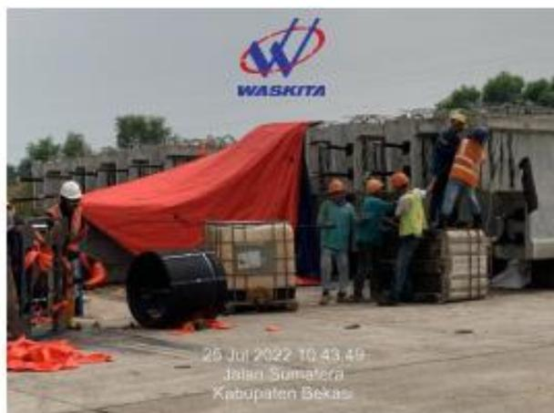
**Gambar 4.8** Proses *Stressing Girder*
