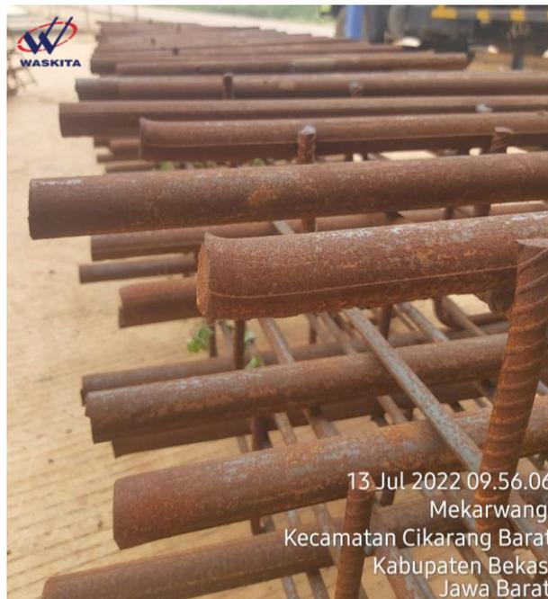
**Gambar 2.4** Tulangan Dowel Diameter 32 mm
