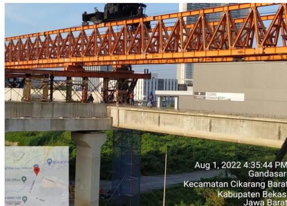
**Gambar 2.27** *Placing Girder ke Bearing Pad*
