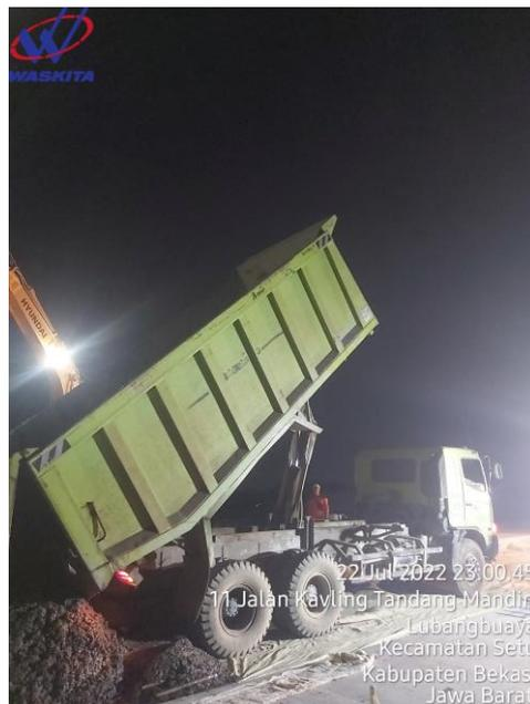
**Gambar 4.5** *Dump Truck* Menuangkan Beton Kelas P (K450)
