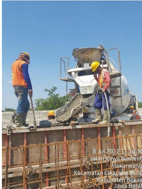
**Gambar 4.18** Proses Pengecoran Parapet
