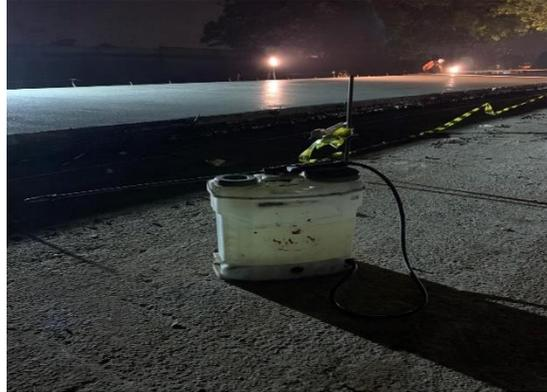
**Gambar 3.6** Alat Curing Manual
