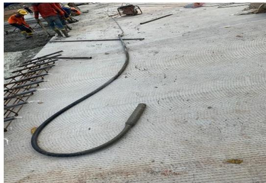
**Gambar 3.4** *Vibrator Concrete Machine*
