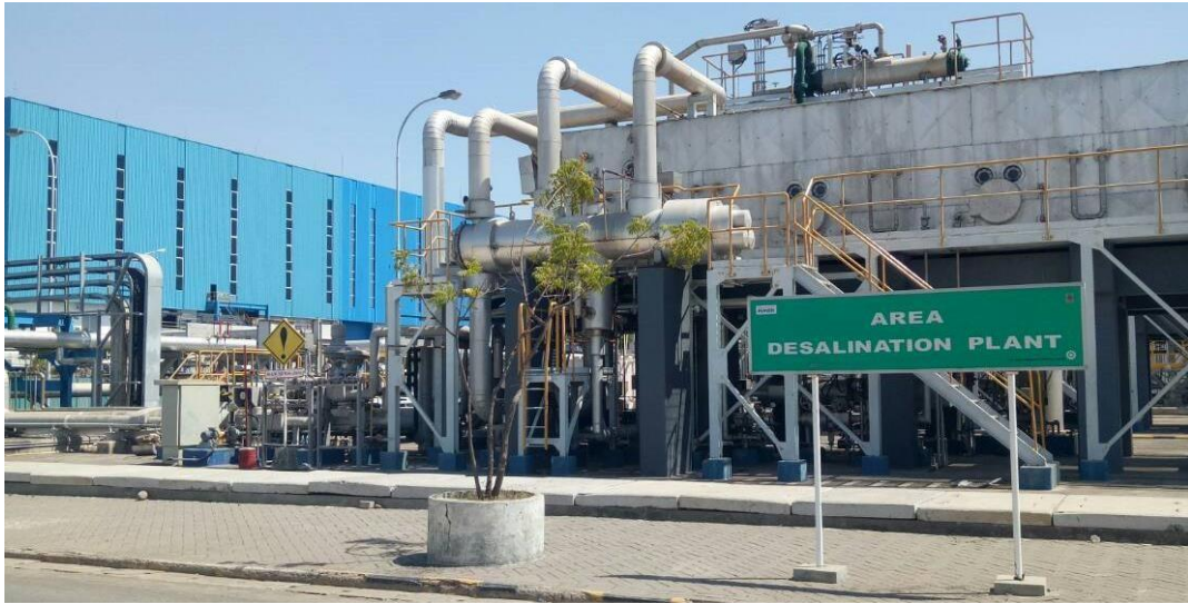
Gambar 4.18 Area Desalination plant
