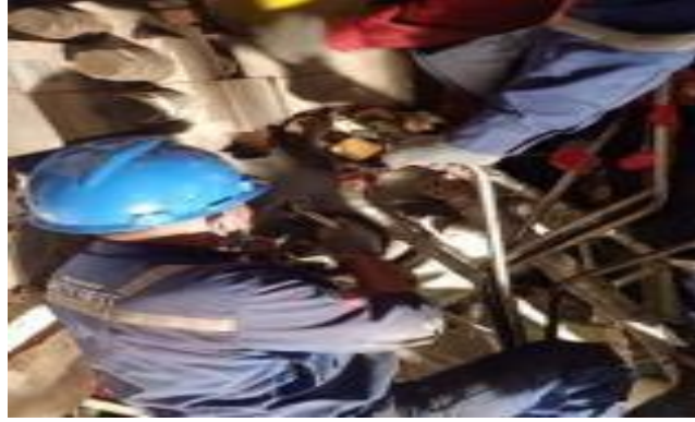
Gambar 4.27 Pelepasan Oil Pipe & Gas Pipe
