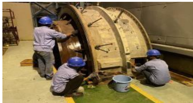
Gambar 4.33 Pembersihan upper exhaust cylinder
