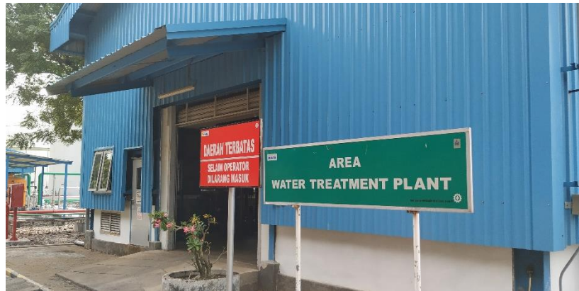
Gambar 4.19 Area water treatment plant
