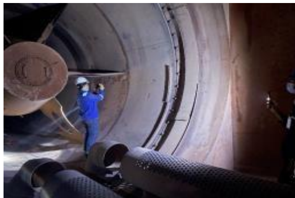
Gambar 4.31 Inspeksi didalam exhaust manifold
