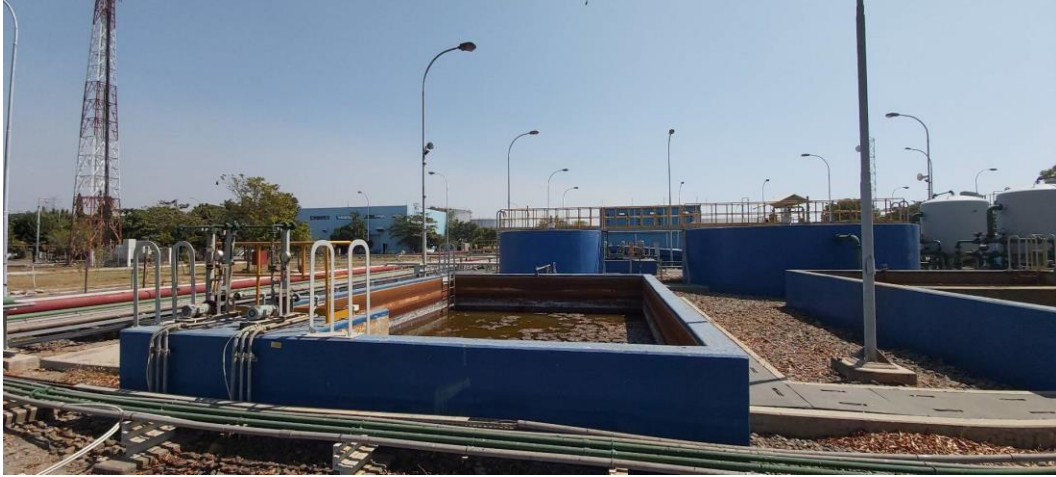
Gambar 4.20 Area Waste Water treatment plant
