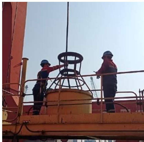
d) Greasing kabel headblock
