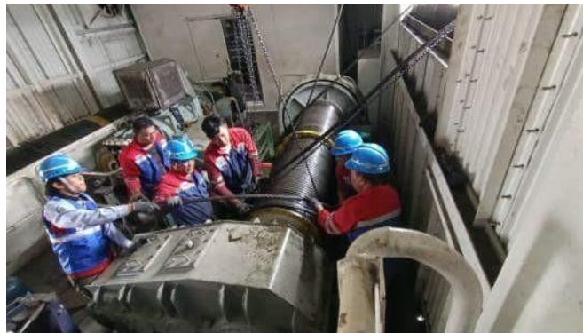
d) Greasing kabel headblock
