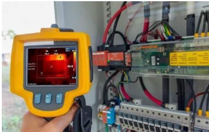
Gambar 4.50 Proses infrared thermography
