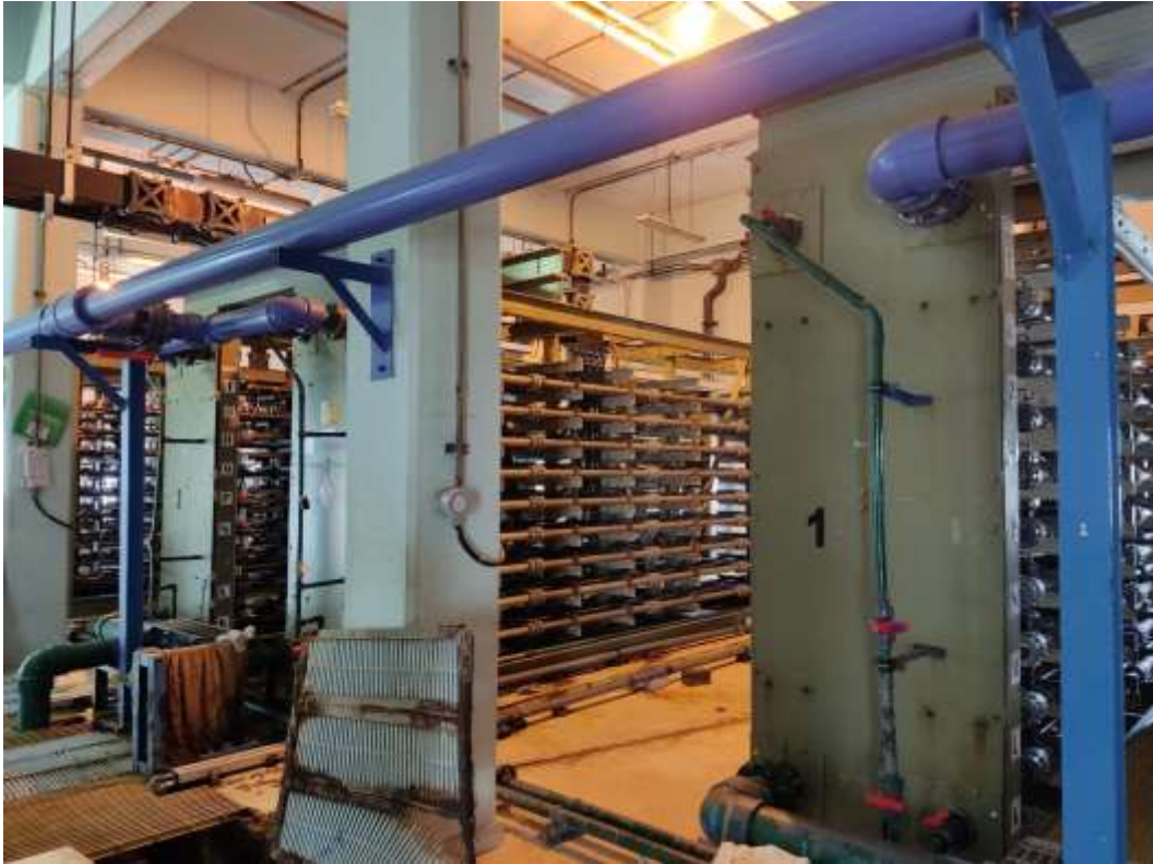
Ruangan Clorination Plant
