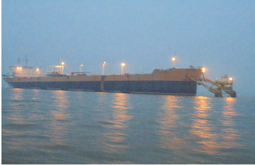
Gambar 3.2 mooring wishbone arm system attach to tripod SPOLS (Single Point Offshore Loading System) (Sumber ;PT. Energi Mega Persada, 2014)
