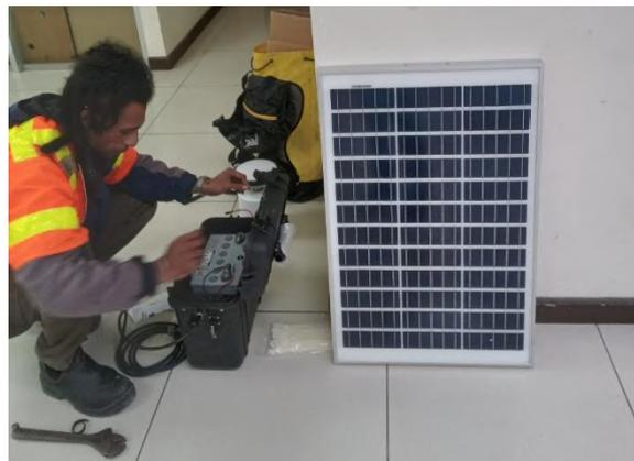
**Gambar 2. 15** Instalasi GPS ke *Power Supply*
