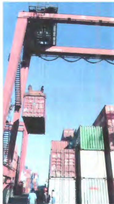
Gambar 2.14. Rubber Tyred Gantry
