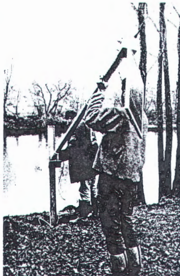
... insert pole with solar panel and GSM antennae into the stand ...
