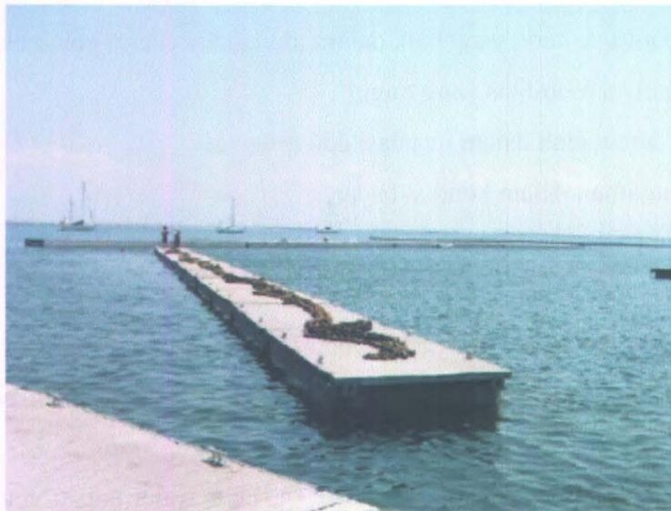
Gambar 2.1 *Concrete Floating breakwater* (FDN,2005)
