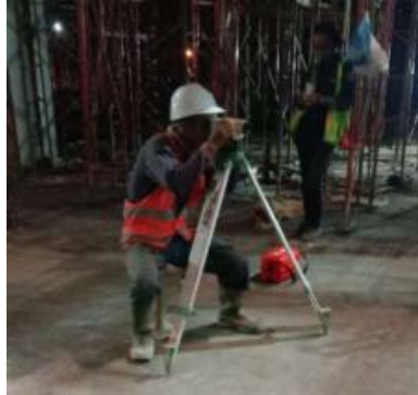
Gambar 5.2 Menentukan As Kolom atau Marking As
