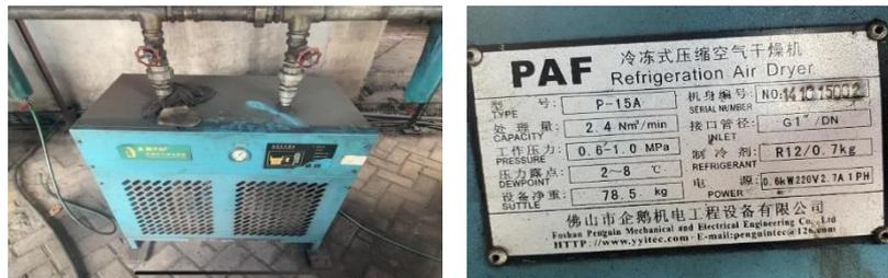
*Gambar 4.35 Refrigeration Air Dryer*
