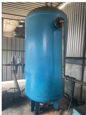
*Gambar 4.37 High Pressure Air Receiver Tank*
