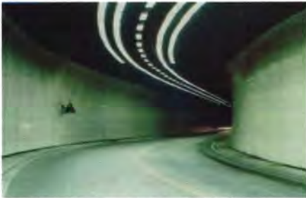
Gambar 2.2: Felbertauern Road Tunnel
