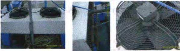
*Gambar 4.4 Kondensor system RSW KM Napoleon*
