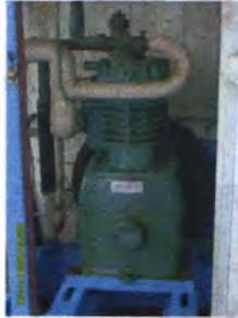
*Gambar 4.3 Compressor system RSW KM Napoleon*
