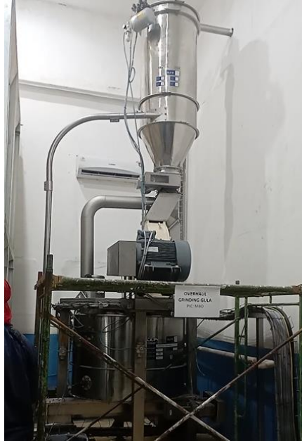
Gambar 4.24 Proses Over Haul Mesin Grinding Gula
