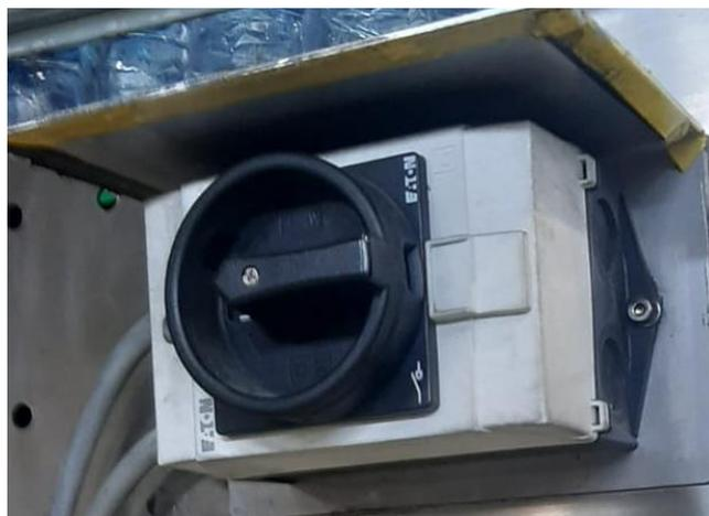
**Gambar 4.28** Switch ON/OFF
