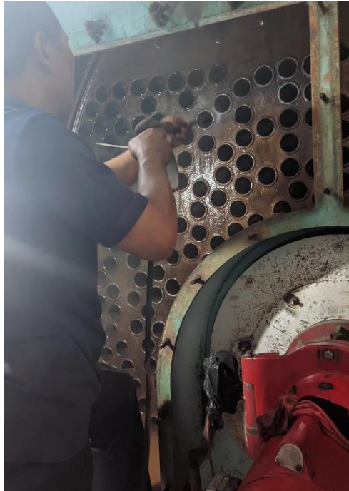
Gambar 4. 16 Boiler Cleaning
